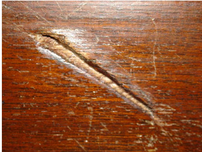
A crack in the wood paneling of a second-storey wall caused by a glass shard.
